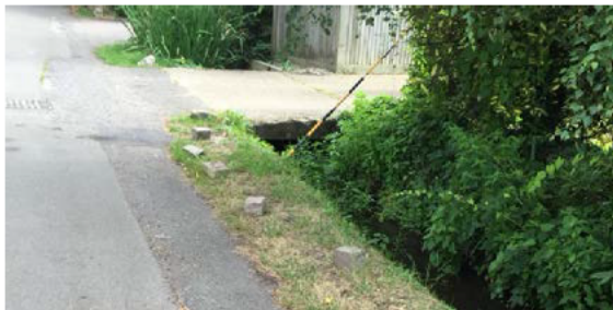
A) INFILLED AND UNDERSIZED OR OVERGROWING CULVERTS ALONG CHAPEL LANE
