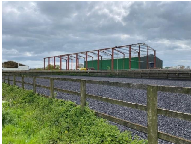
Photo 1: The Manege, Temp Building 1, steel frame of Building 7, and Building 8
