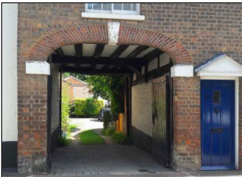
Timber frame visible in carriage arch to 59 High Street
