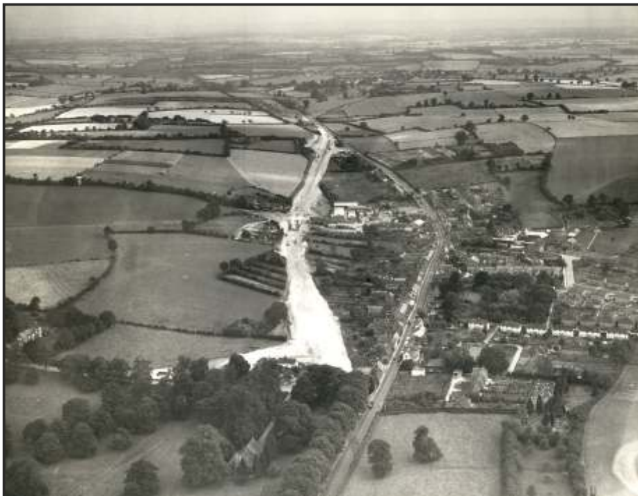
Construction of the Markyate bypass in 1955 showing the chalk revealed by removal of topsoil, aerial view looking south (BEAMS photographic archive)
