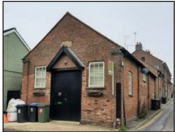
Former Primitive Methodist chapel, corner of Cleveland Road and Pickford Road
