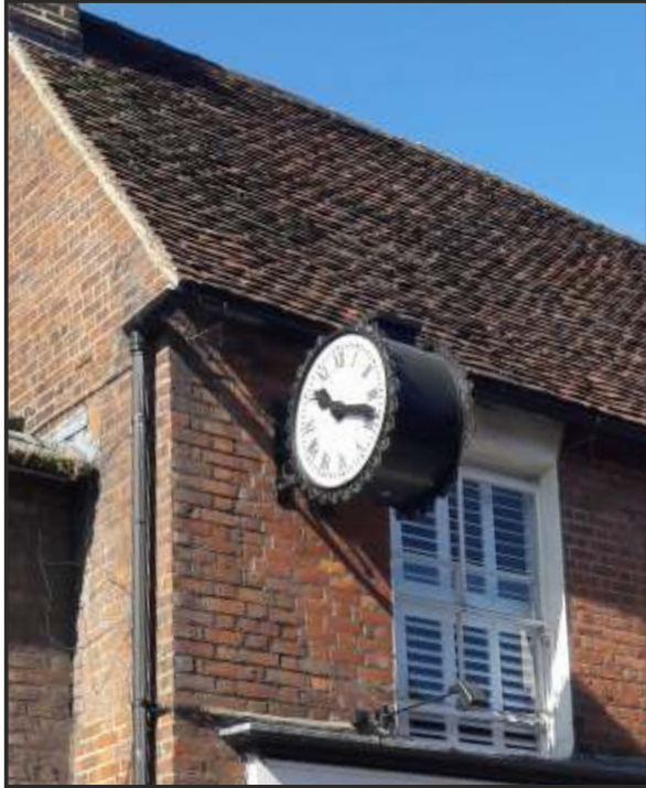
Coronation Clock (1911) attached to the frontage of 48 High Street
