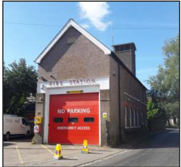
Markyate Fire Station
