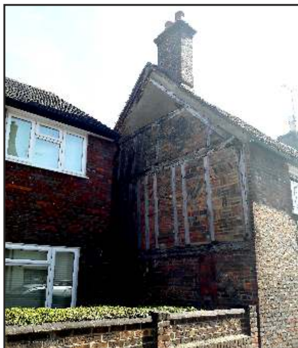
Timber frame to gable end, 117 High Street
