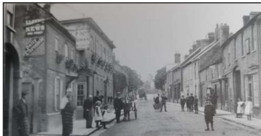
Markyate High Street, looking north with the Swan Inn on the left side
