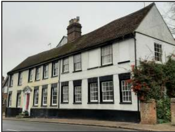
Sash windows to The Grange
