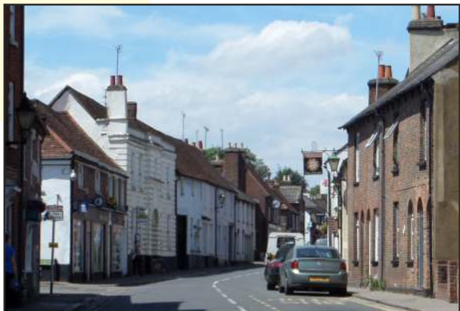
The curve of the High Street, looking north, at the southern end of the Conservation Area
