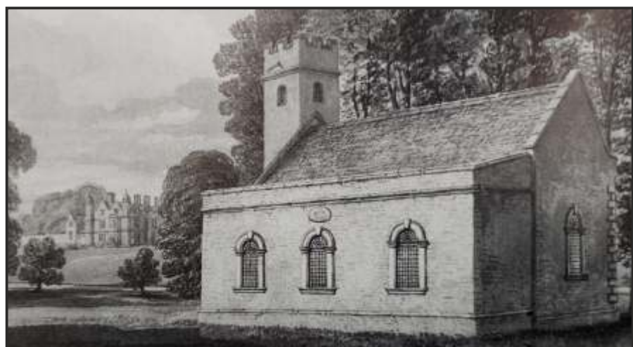
Drawing by Buckler (c. 1830) of St John the Baptist with Markyate Cell in the background (Markyate Local History Society, 2002)
