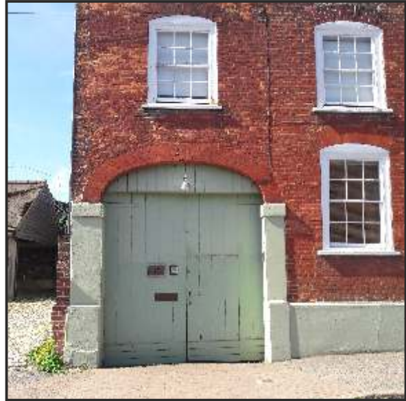
Elliptical carriage arch to Cavendish House
