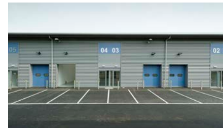
Maylands Business Centre in Hemel provides hot-desking and small-scale office and industrial units plus a business development programme and networking spaces.
