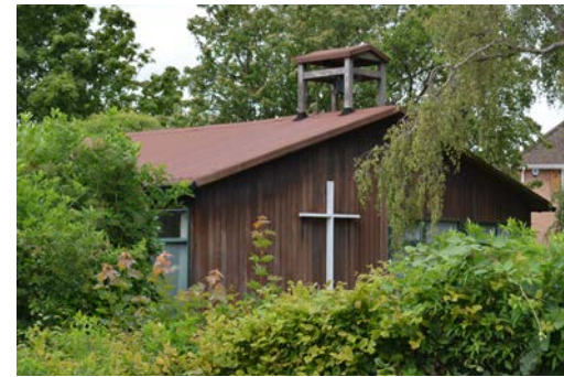
The church of St. Stephen, Hemel Hempstead (1959) was designed such that it can be converted from church to community room simply by sliding a screen.
