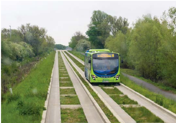
The Cambridgeshire Guided Busway connects Cambridge, Huntingdon and St Ives. In the first year of operation 2.5m trips were made. The busway integrates green infrastructure along its length.
