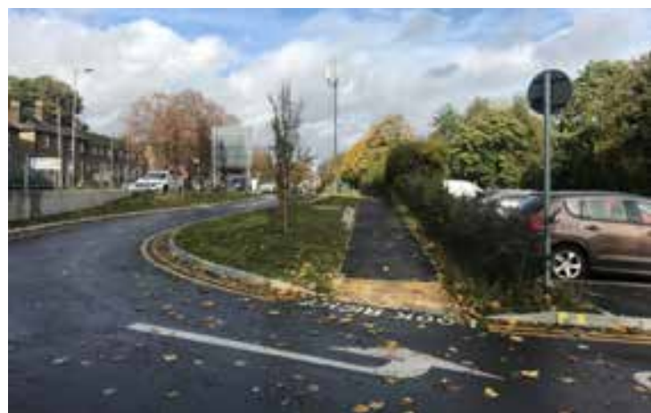
Entrance to the Water Garden Car Park South from Leighton Buzzard Rd
