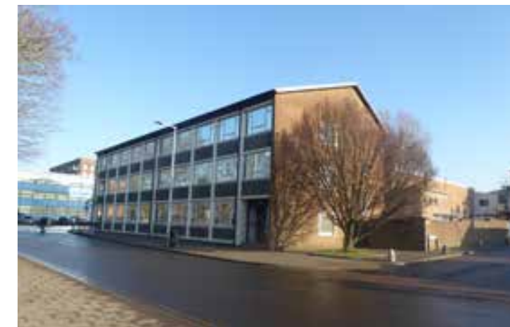
View of Job Centre
