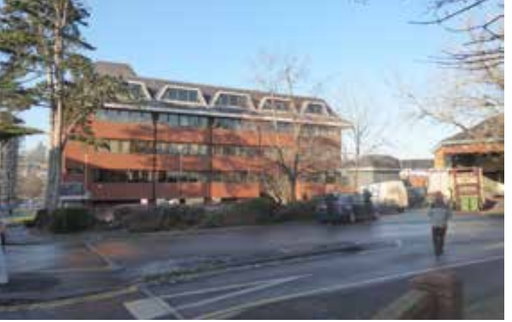
View of the office building from Hillfield Road looking west
