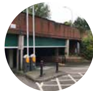
2. WATER GARDENS CAR PARK NORTH
