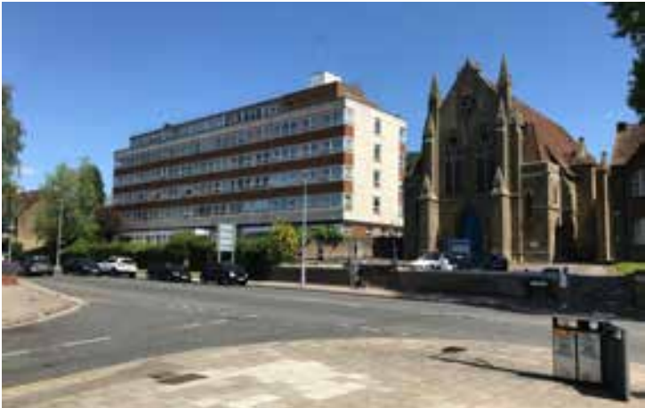
View of Carey Baptist Church located opposite to the Civic Zone site
