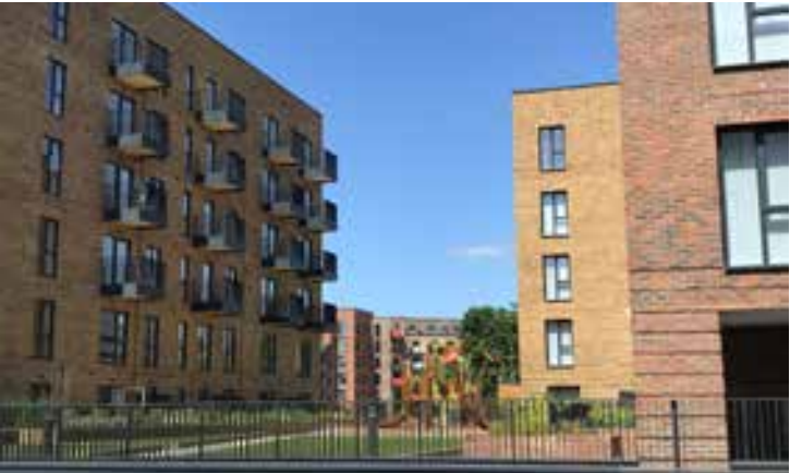
The Gade residential development located on the southern side of the Civic Zone site
