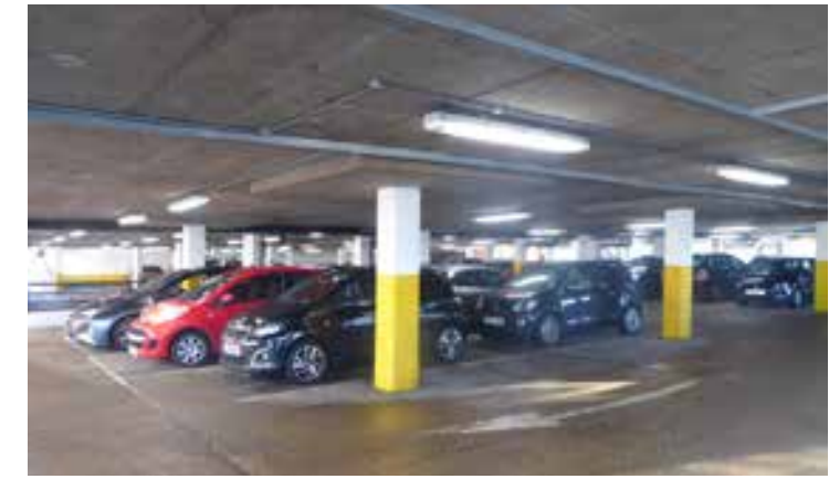
Internal view of the NCP car park
