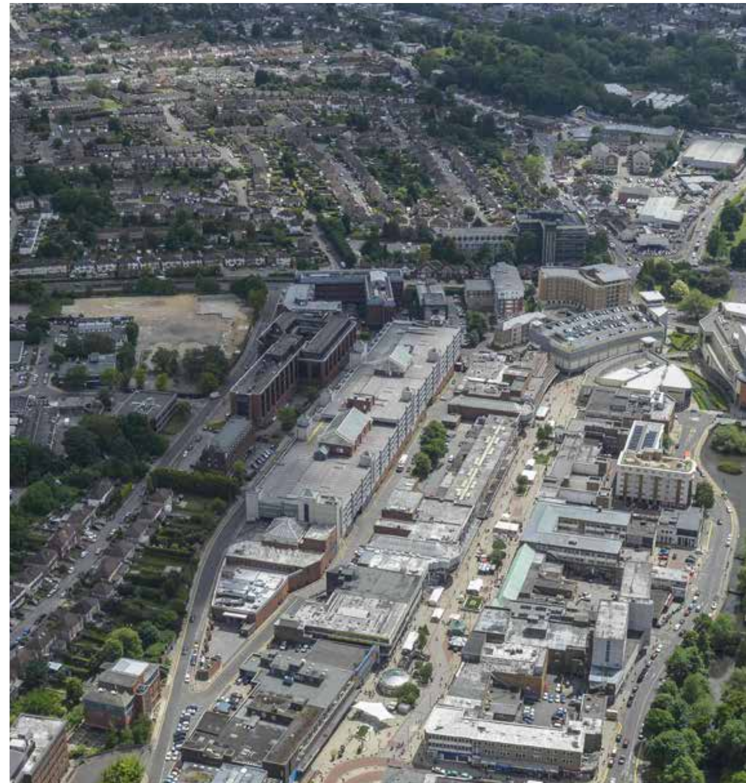
Aerial view of the Marlowes Shopping Centre
