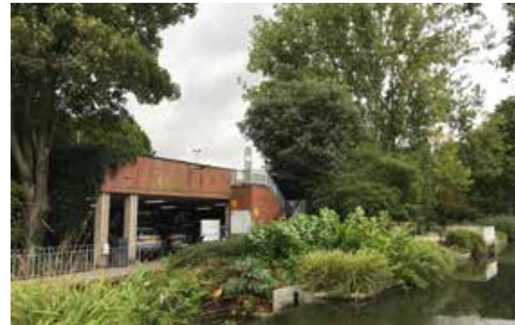
View of Water Garden Car Park North from Bridge Street
