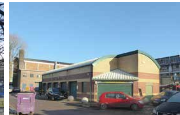
View of Market Square service yard
