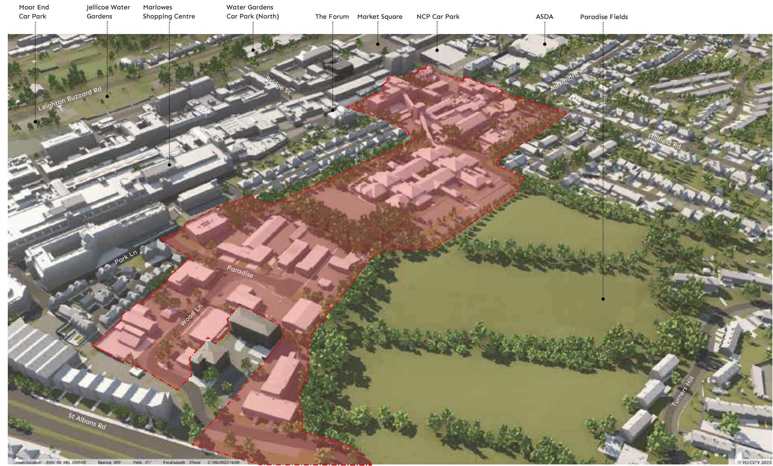
Hospital and Paradise site aerial view extracted from Hemel Hempstead 3D model produced by Vu.City
