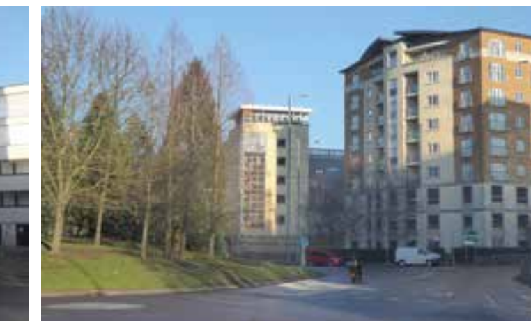
View of Riverside Shopping Centre from the Plough Roundabout looking north
