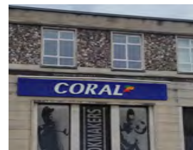
Flint panels and stonework
