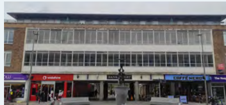
Horizontal rhythm of façade emphasised by projecting eaves of oversailing flat roof
