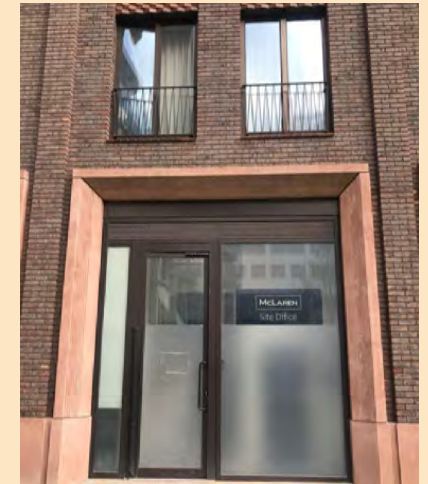
Saxon Court uses secondary elements to reinforce entrances and windows
