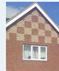
Red & buff brick characteristic of many of the recent developments
