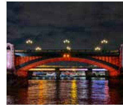
Image of Southwark Bridge
