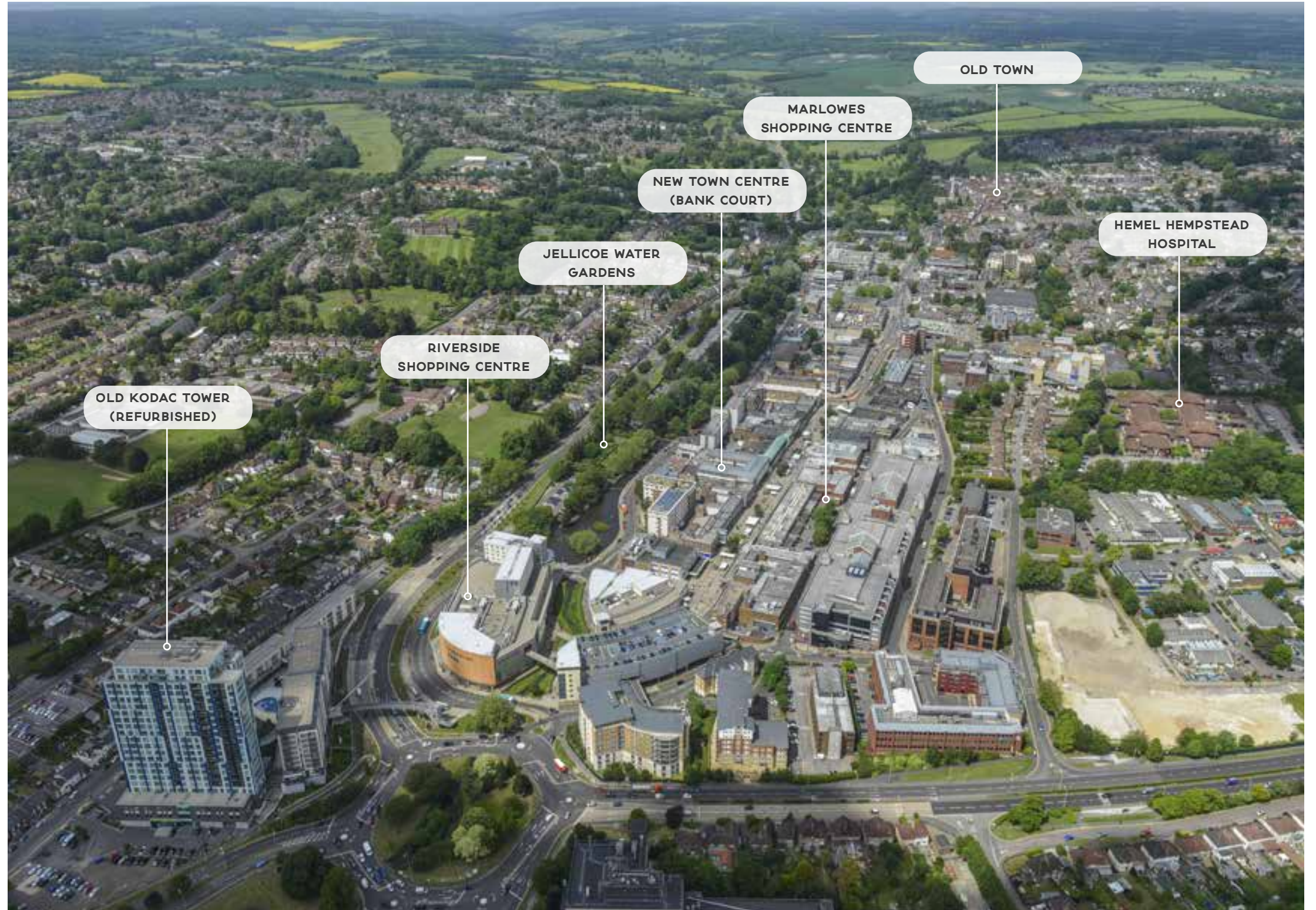
aerial view of Hemel Town Centre
