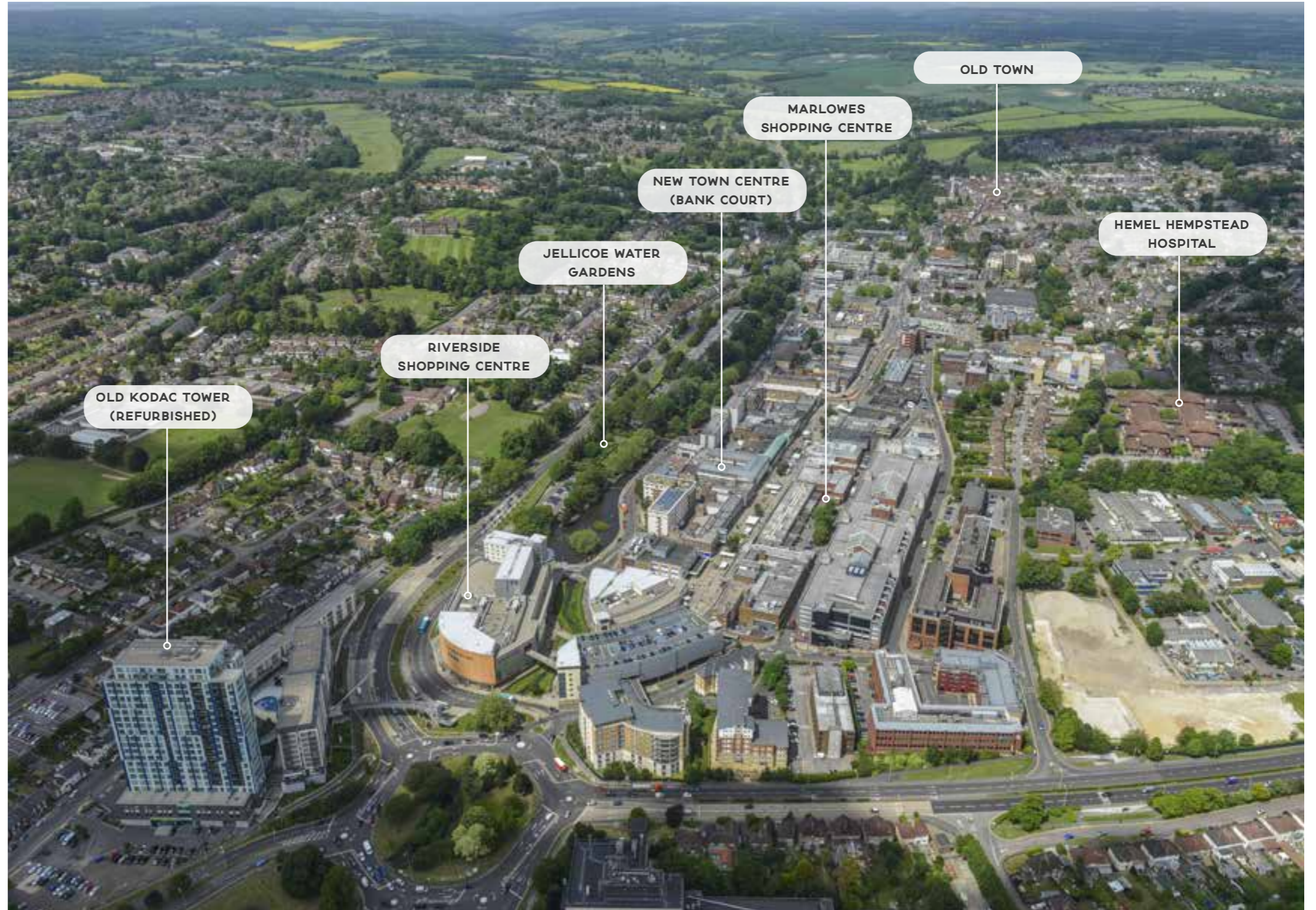
aerial view of Hemel Town Centre
