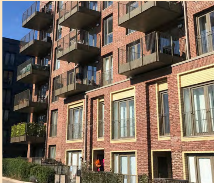
This block in Burrige Gardens demarcates windows using a different tone of brickwork and uses different balcony extrusions to add interest
