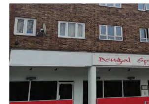
Framing of shopfronts and windows with contrasting surrounds
