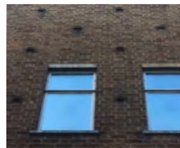
Buff brick with textured brickwork
