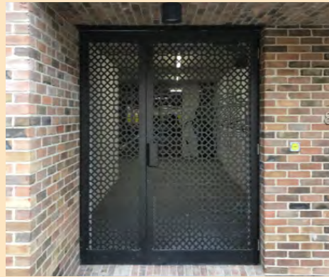
The entrances to the homes within the Colville Estate use lattice detailing on the doors which complements the brick façade
