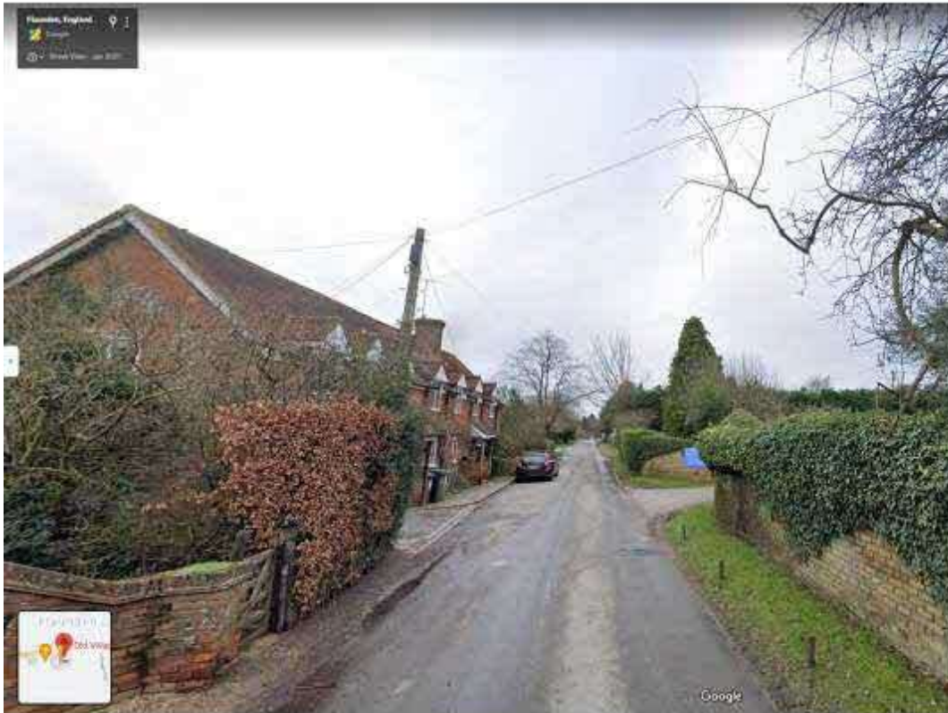
Lack of public pavement across the house frontage and no public paving on the other side of the road (Old Village Hall located on the left)
