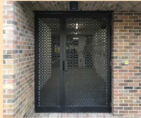
The entrances to the homes within the Colville Estate use lattice detailing on the doors which compliments the brick façade
