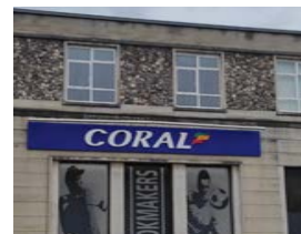
Flint panels and stonework
