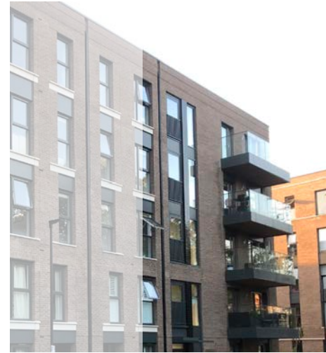
Partially inset balconies are considered a more sustainable option to inset balconies whilst maintaining a clean and simple façade.
