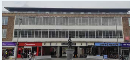
Horizontal rhythm of façade emphasised by projecting eaves of oversailing flat roof
