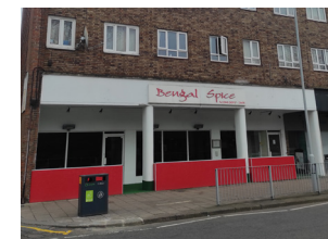
Strong framing of shopfronts and windows
