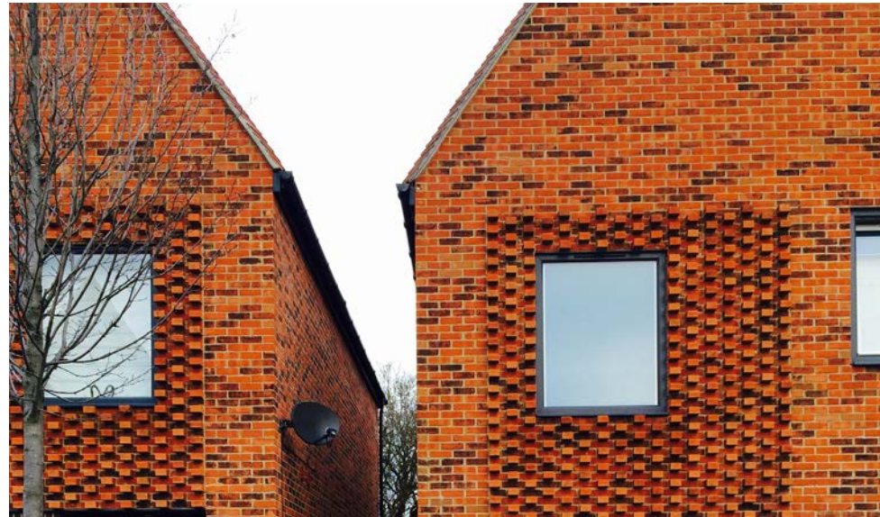
Textured brickwork is used to add interest to the façade in Horsted Park.
