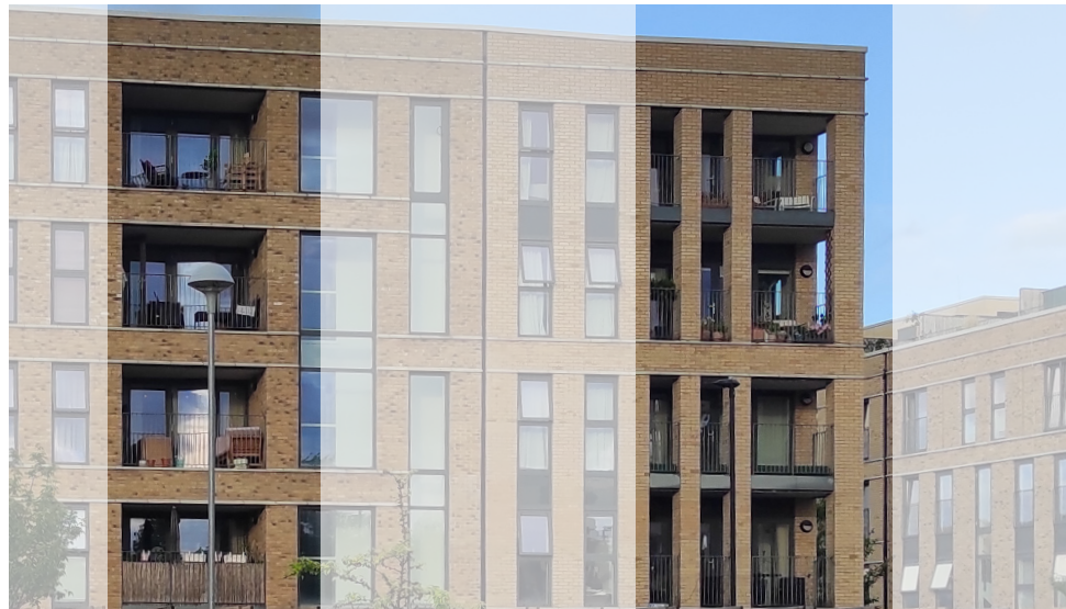
Inset balconies are an option on south facing units, or units overlooking Paradise or Wood Lane
