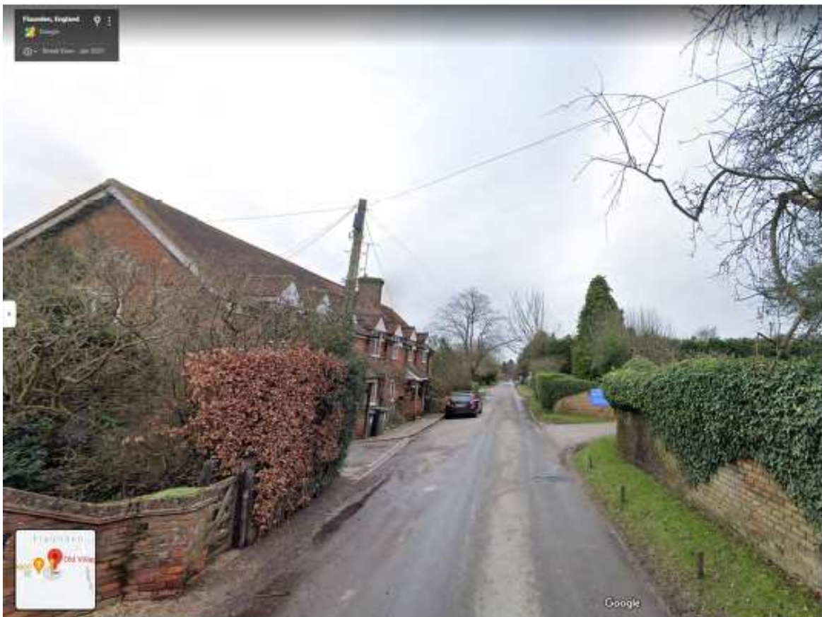
Lack of public pavement across the house frontage and no public paving on the other side of the road (Old Village Hall located on the left)
