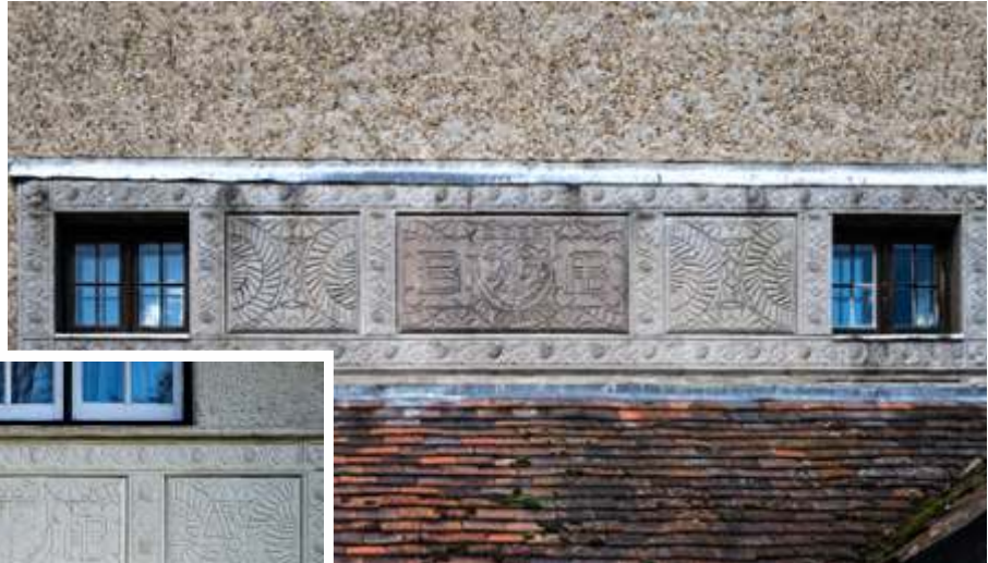
Render and pargetting to No 20 (left) and No 21 (above)
