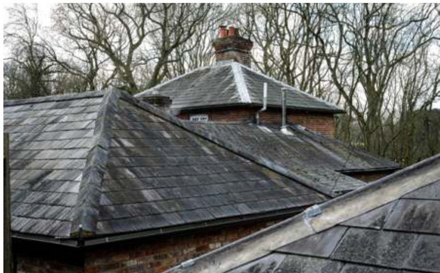
Home Farm slate roofscape
