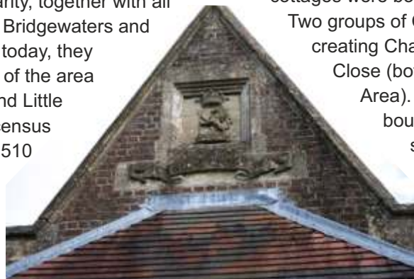
Shield on front wall of Little Gaddesden House
