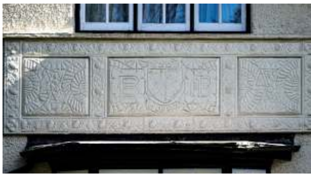
Render and pargetting to No 20 (left) and No 21 (above)
