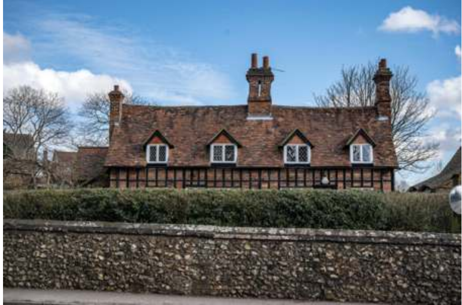
No 22/23: Timber-framing, infill brickwork, peg tiles and leaded light casement windows. Front boundary flint wall and hedging.
