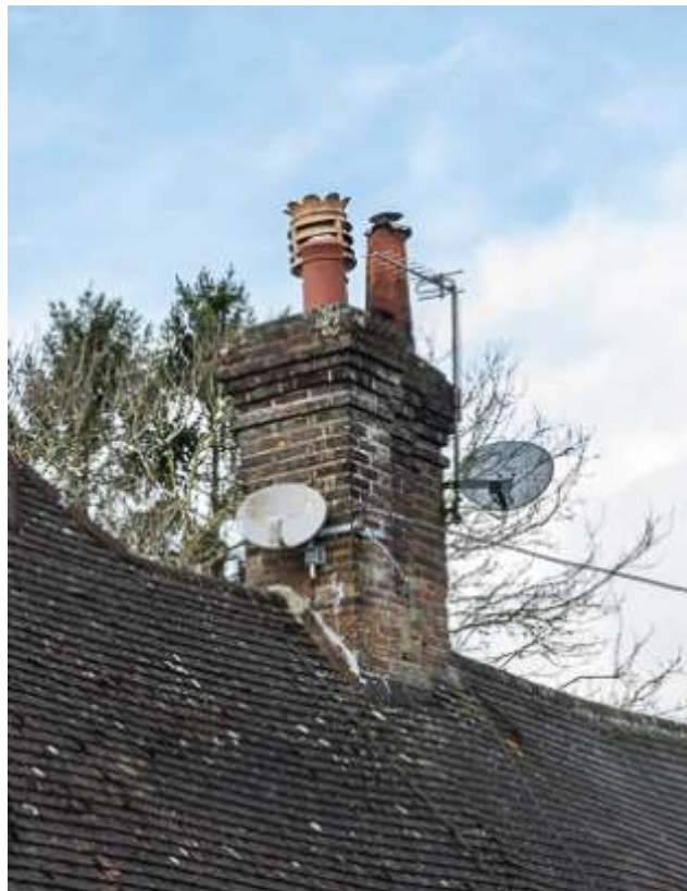
15-17 close up of satellite dishes
