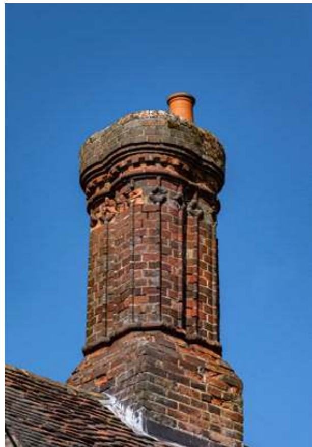
Decorative chimney at No 42 on the Green
