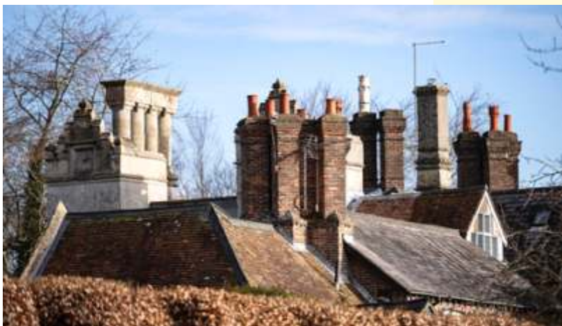
Roofscape of chimneys at the Manor House
