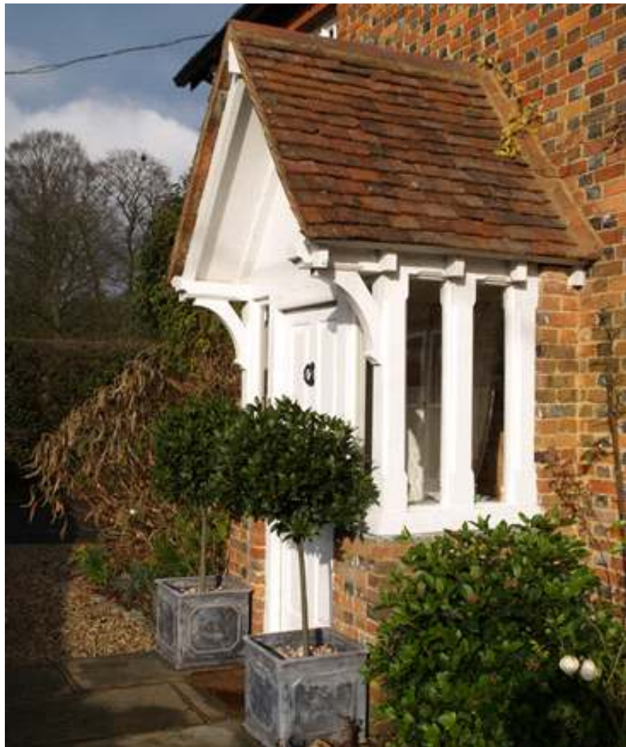
Porch at Keepers Cottage
