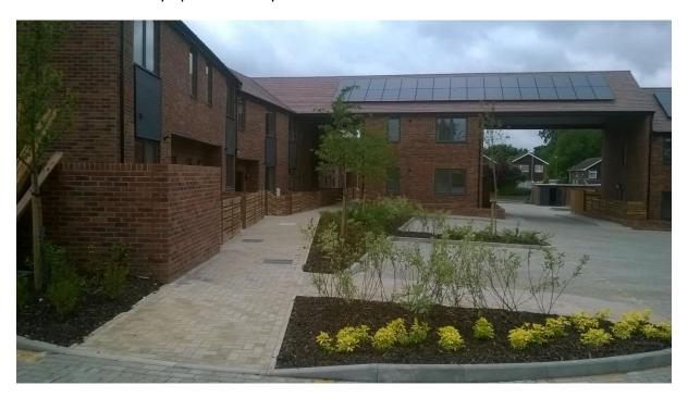
Where appropriate solar PV or solar thermal has been fitted to the new build schemes to generate energy for the communal facilities, as shown above in the image of Farm Place in Northchurch.
