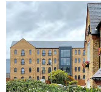
Magenta Court, Apsley, new social rent housing drawing on the area's canalside location and industrial heritage.
