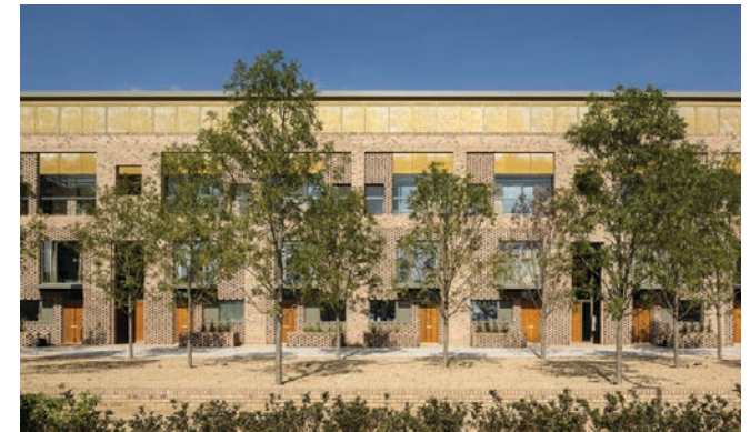
Abode, Cambridge. Proctor & Matthews Architects. Photo: Tim Crocker
