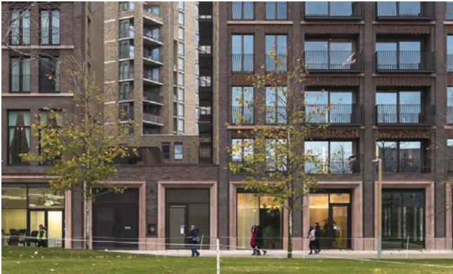
Fenman House, Camden, Maccreeanor Lavington. Photo: Tim Crocker
