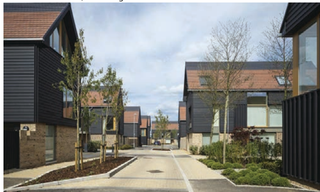
Abode, Cambridge. Proctor & Matthews Architects. Photo: Tim Crocker
