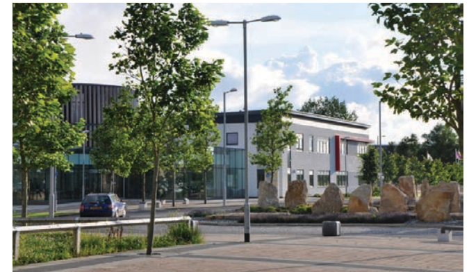
The Enterprise Centre in Priors Hall, Corby
