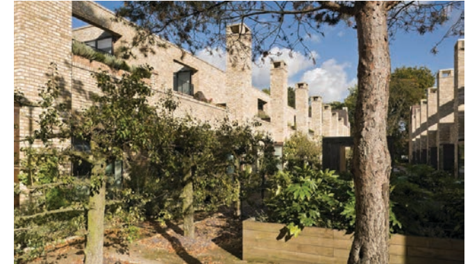
Accordia, Cambridge. Feilden Clegg Bradley. Photo: Tim Crocker
