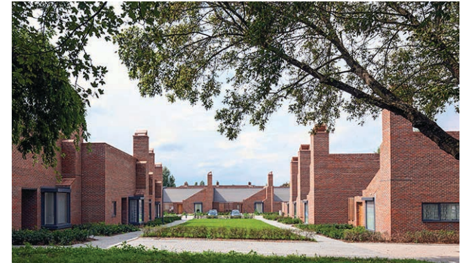
Courtyard Housing, Barking. Patel Taylor. Photo: © Patel Taylor
