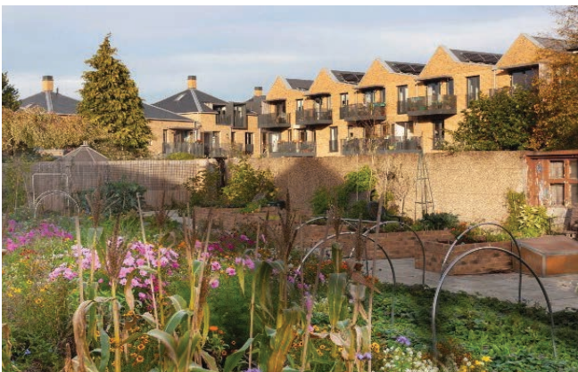
New Ground co-housing, High Barnet
