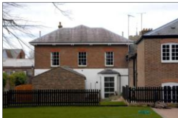
Rear extension to 20 High Street
