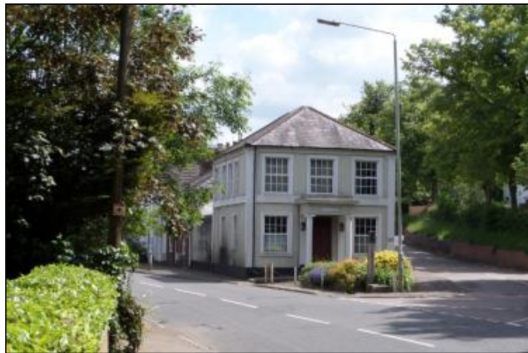
Norfolk House, this property occupies a prominent corner position at the point where Park Road and Western Road meet and is at the entrance to the conservation area from the west
