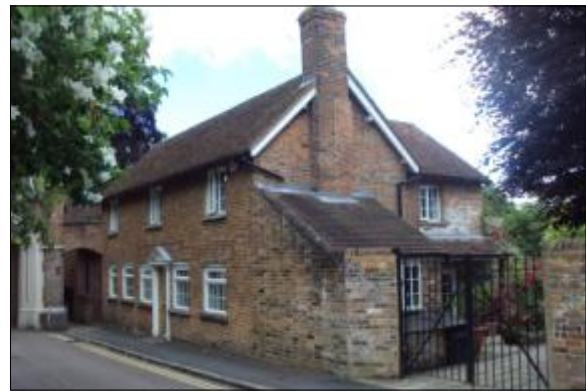
uPVC windows in Vicarage Lodge, Churchyard
