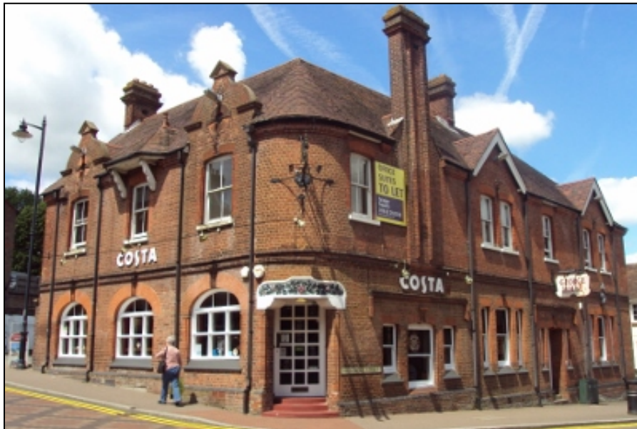
George House on the corner of High Street and Frogmore Street
