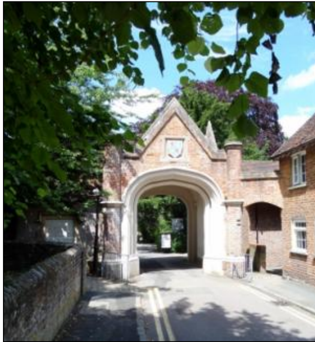
The Gatehouse to Sutton Court, Church Yard
