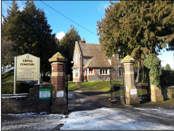
Entrance gates to Tring Cemetery and cemetery lodge
