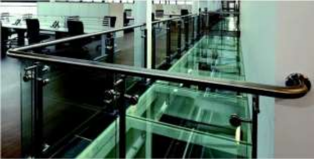
Cat A balustrade.
