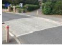
Proposed crossing and signpost feature to improve level of sight lines, encourage vehicles to slow down while also retaining the green lane character.
