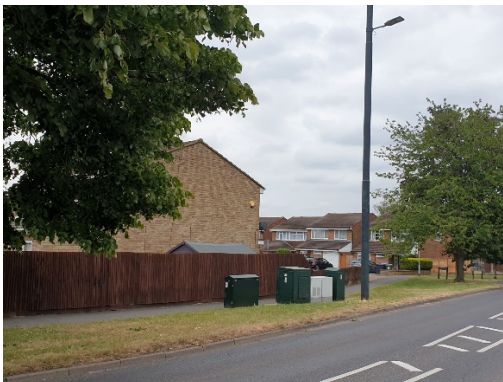
View of Perry Green Existing Mast Mast side view
