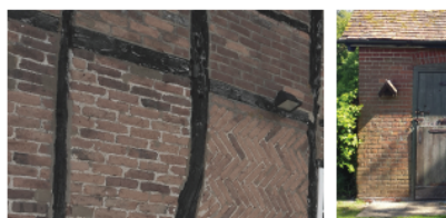
BRICKWORK TO EXISTING BUILDINGS
