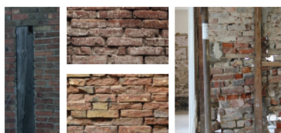
BRICKWORK TO EXISTING BUILDINGS
