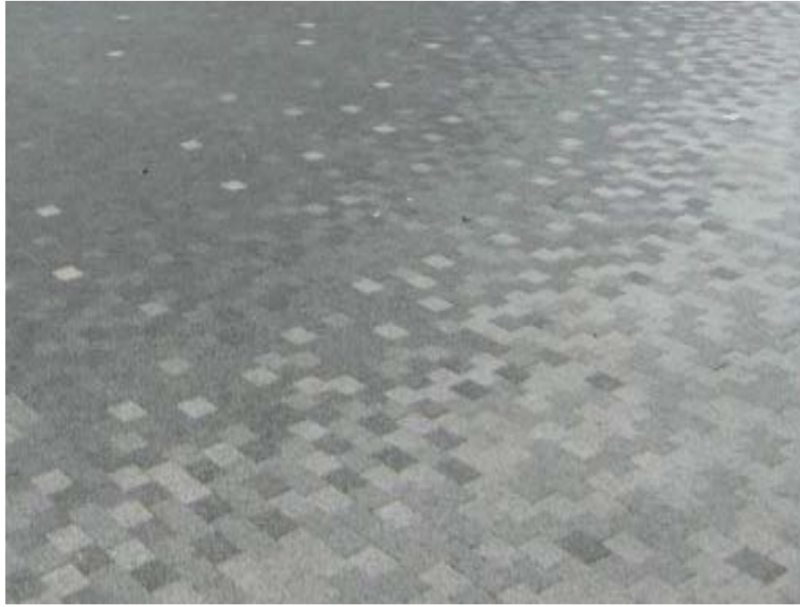
Granite proposed for Water Feature area and Town Square - example of feathered pattern
