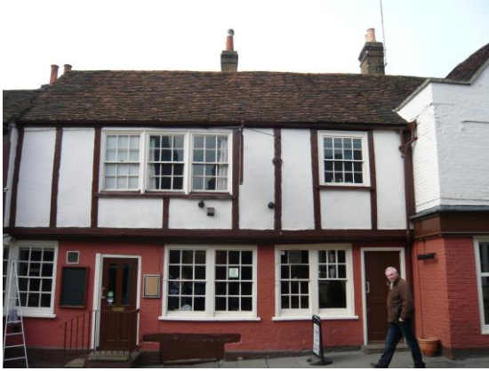
Figure 10: The use of the sash window is a unifying characteristic of the conservation area (seen here punched into the facades of an earlier timber framed building – The
