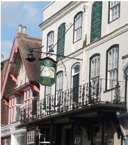
Figure 58: Hanging signage on decorative brackets - The Old Bell, High Street
