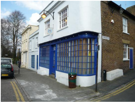
Figure 57: There is a good survival of traditional historic shopfronts
