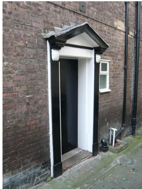
Figure 60: door surround and hood, High Street
