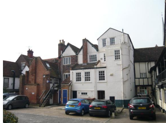
Figure 13: Rear of No.37-39 High Street – typical example of the organic extensions and alterations to buildings fronting the High Street.
