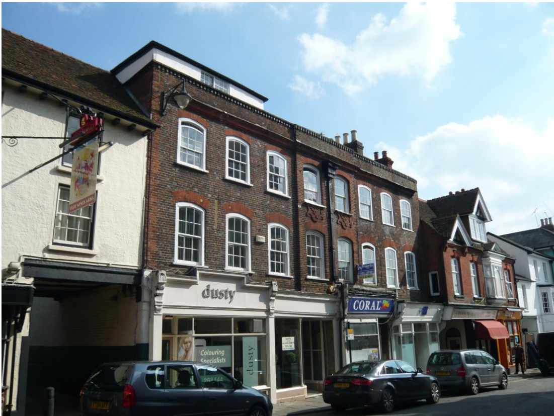
Figure 53: Development of the early 18 th century (dated 1736) with notable use of the cambered head to windows
