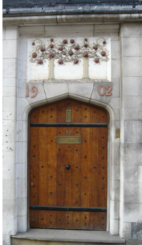
Figure 59: No.28 High Street - mock Tudor door
