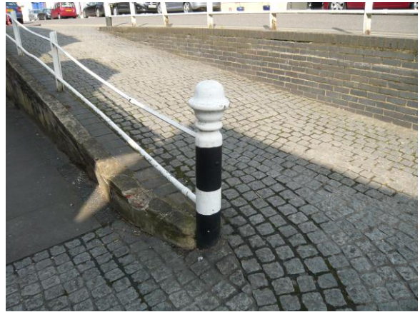
Figure 44: Traditional cast iron black and white stripe bollards to the northern end of the High Street
