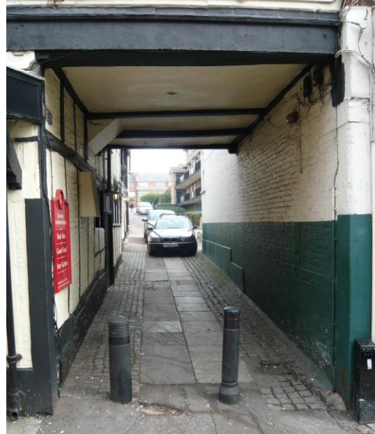
Figure 39: Some enhancement of the floor surfaces has taken place over the years (alley between 39 and 41 High Street)
