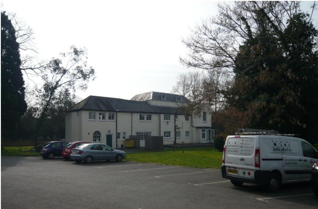
Figure 34: The setting of The Bury is marred by parking
