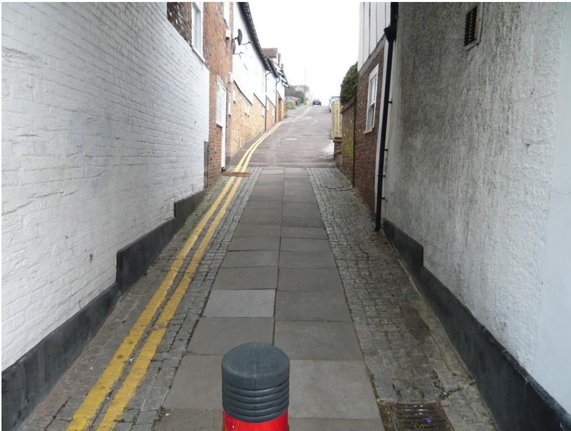
Figure 66: Inappropriate and unnecessary use of double yellow lines in alleyways
