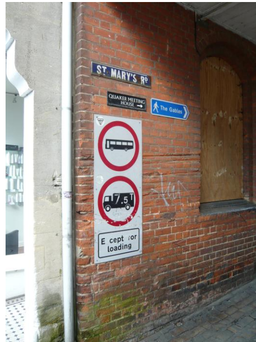
Figure 64: Unnecessarily large and inappropriate signage to the High Street
