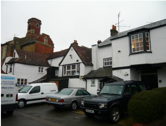
Figure 36: The rear of historic buildings often comprises parking courts or public car parks
