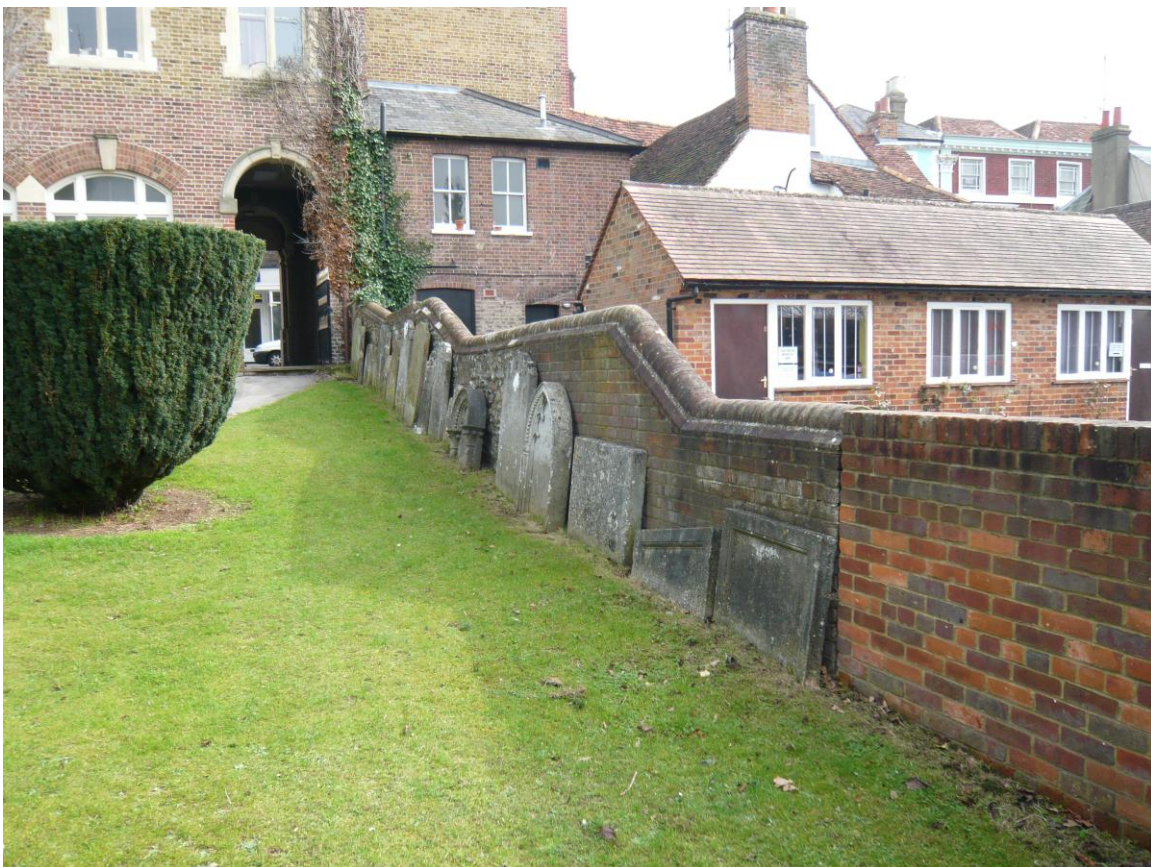
Figure 61: Brick and flint boundary walls are important vernacular features which survive within and to the boundaries of the conservation area
