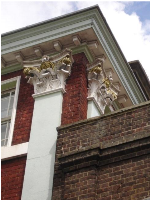
Figure 56: Corinthian pilasters to No.25 High Street
