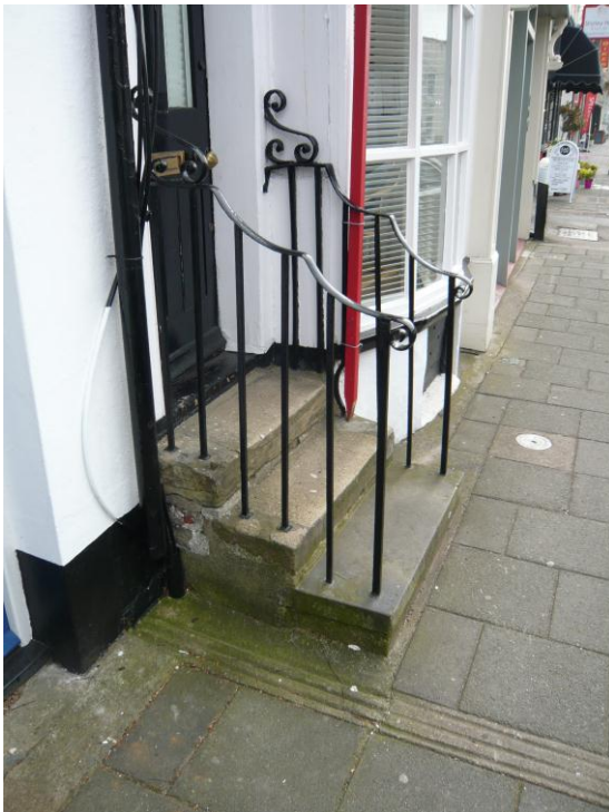
Figure 54: Decorative Wrought iron railings to steps, High Street
