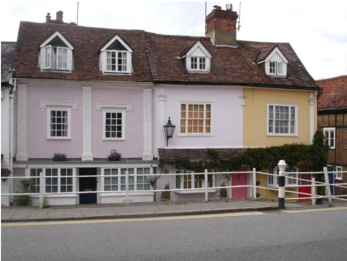
Figure 55: Examples of dormer windows, 68-72 High Street
