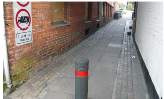
Figure 40: Granite setts to gulleys survive to some of the lanes and alleys (many have been replaced or relaid) (alley between 51 and 53 High Street)
