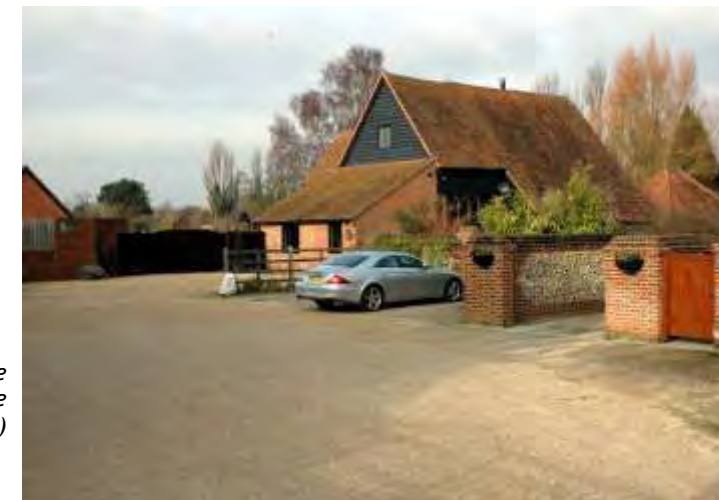
More traditional surfacing materials have much less impact and are usually more permeable. (Little Missenden)
