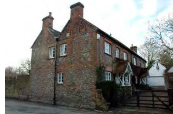
The roof of this relatively large cottage is kept in proportion by the use of a double roof with central valley gutter. (Coleshill)
