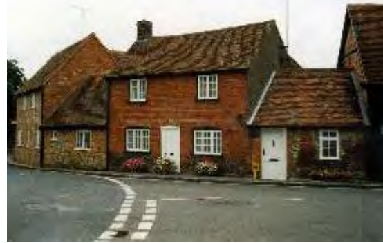
The buildings fit together because the roof pitches and use of plain red clay tiles is consistent. (Little Missenden)
