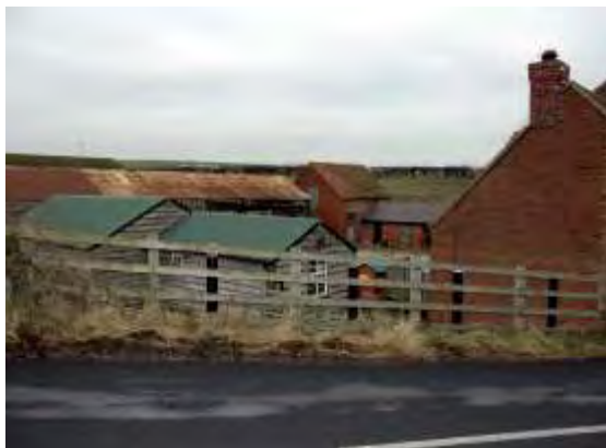
A more appropriate colour on the roofs would have helped these new buildings integrate more effectively. (Little Tring)
