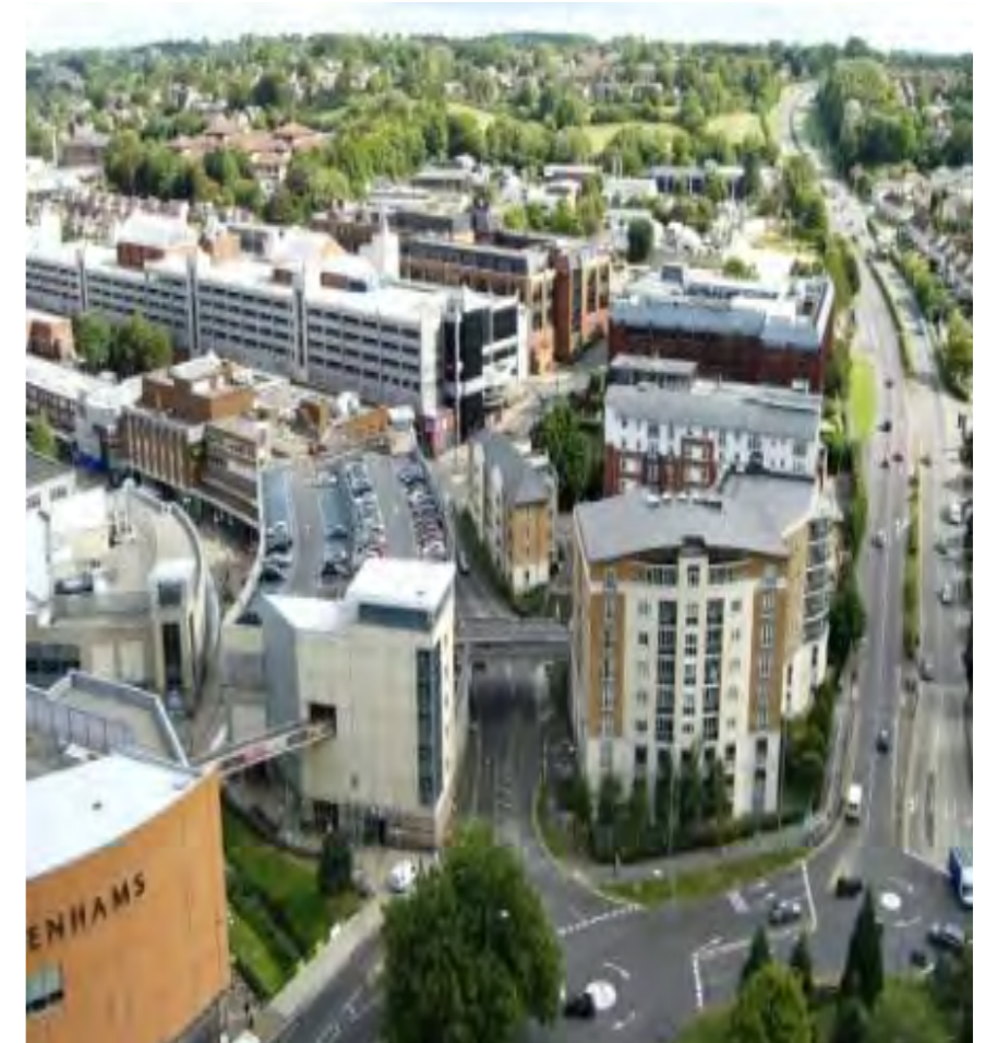
View of Plough Roundabout - access and movement (Source : DBC)
