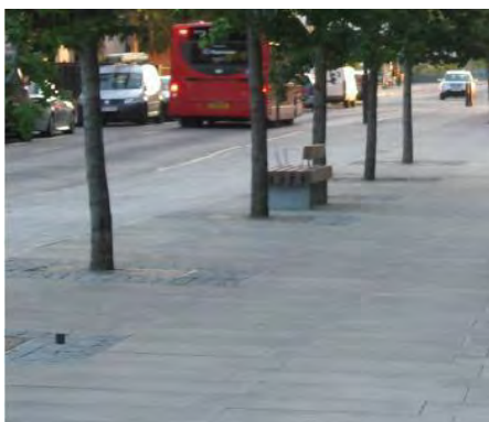
High quality concrete paving
