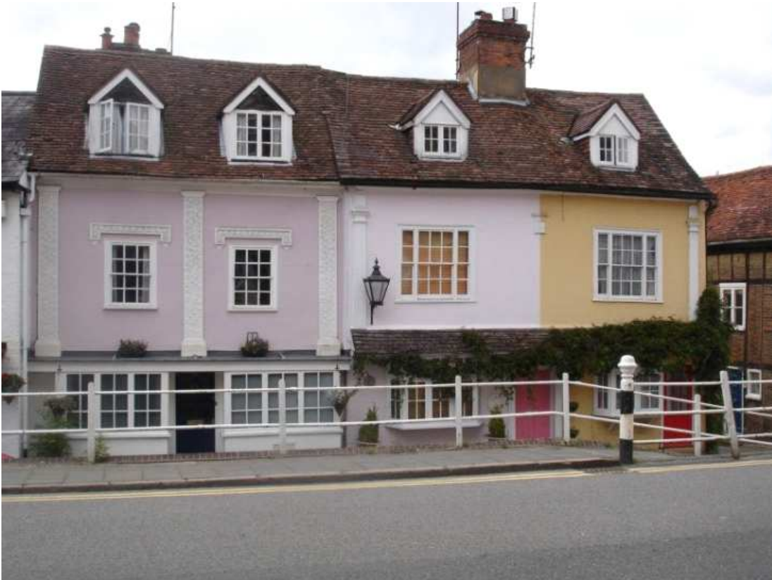
Figure 52A: Examples of dormer windows, 68-72 High Street
