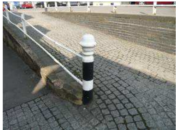
Figure 42A: Traditional cast iron black and whiter stripe bollards to the northern end of the High Street
