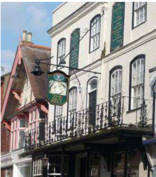
Figure 52D: Hanging signage on decorative brackets - The Old Bell, High Street
