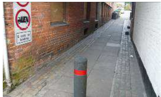
Figure 40: Granite setts to gulleys survive to some of the lanes and alleys (some have been replaced or relaid) (alley between 51 and 53 High Street)
