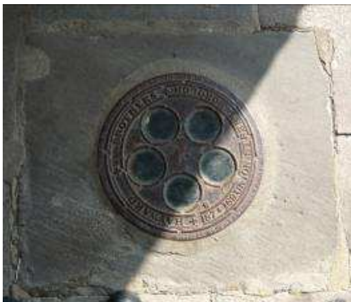
Figure 41A: A early 20 th century cast iron inspection cover
