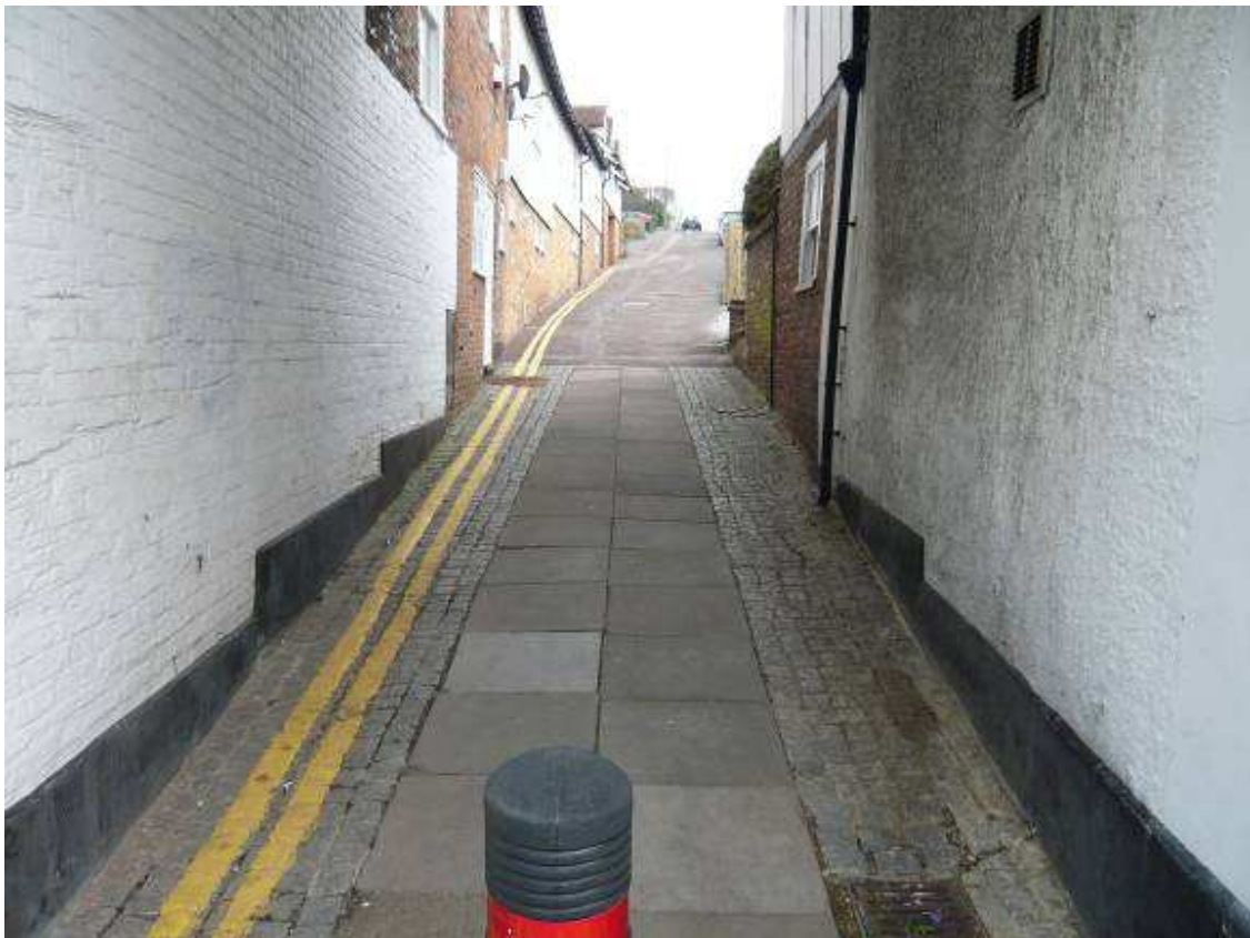
Figure 57: Inappropriate and unnecessary use of double yellow lines in alleyways
