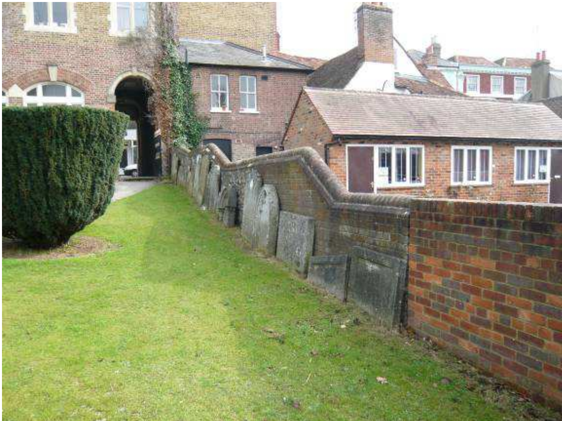
Figure 53: Brick and flint boundary walls are important vernacular features which survive within and to the boundaries of the conservation areas
