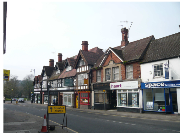
Figure 44: Built form to Queensway generally a mix of two and two and a half storey shops with accommodation above (some upper floors are used as offices)
