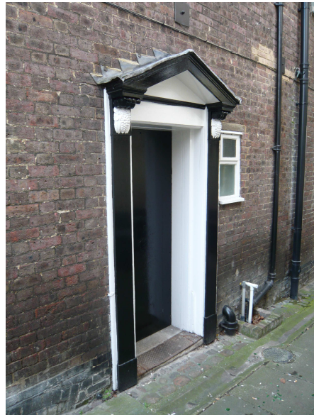
Figure 52F: door surround and hood, High Street
