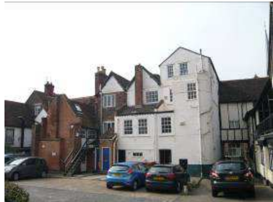
Figure 13: Rear of No.37-39 High Street – typical example of the organic extensions and alterations to buildings fronting the High Street.
