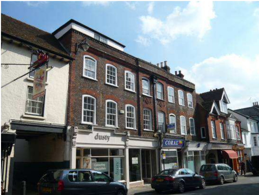
Figure 51: Development of the early 18 th century (dated 1736) with notable use of the cambered head to windows
