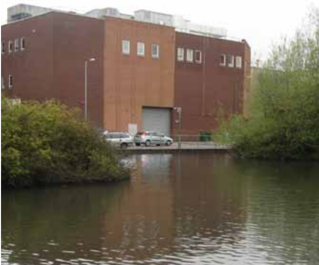
Loss of positive frontage on adjacent buildings
