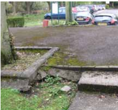
Footpath surfacing replaced with macadam. Brick edging to tree surrounds
