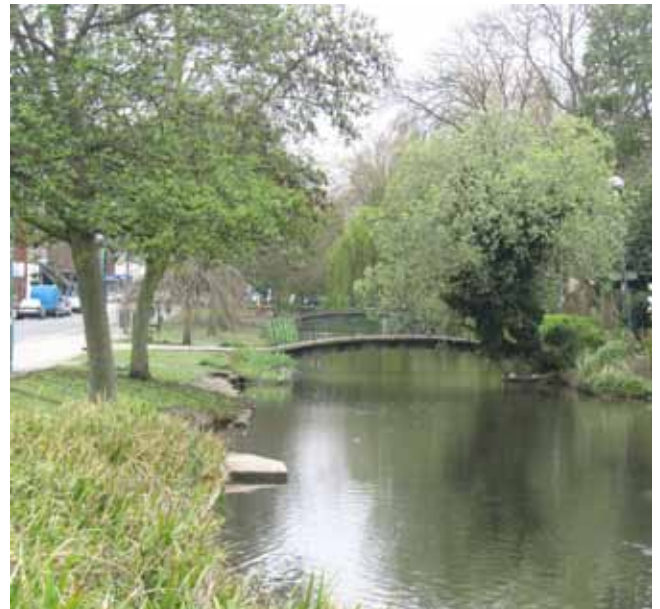
Eroded banks detract from the canal effect
