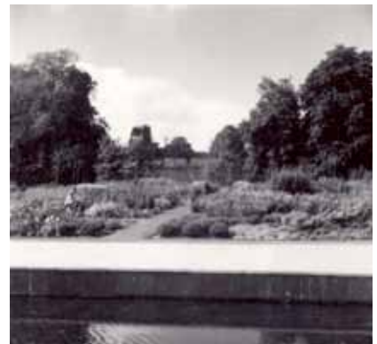
Flag paving overhanging revetment
