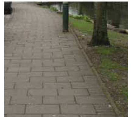
Large format paving flags without edgings have been replaced with smaller units, with brick detailing and concrete edging
