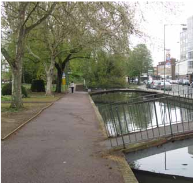
Flag terraced reduced in width, resurfaced in tarmac and brick coping introduced
