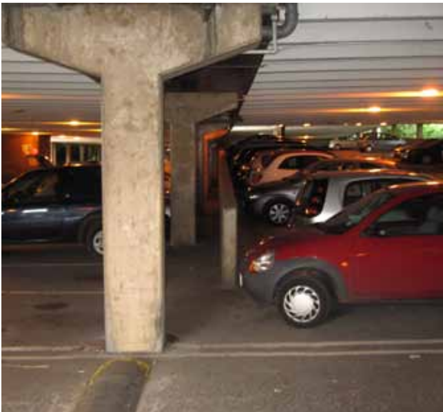
Photograph showing start of retaining wall at base of ramp to upper deck
