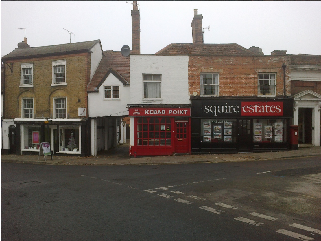
Front of premises
