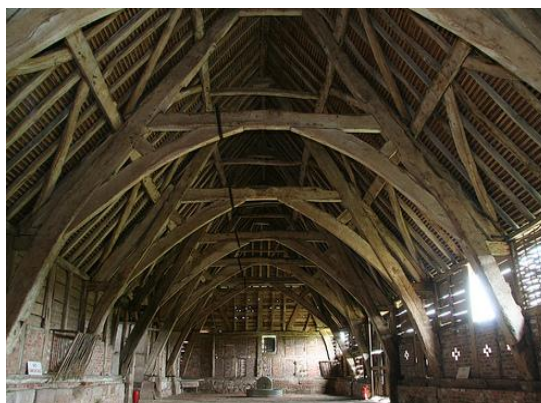
Tithe Barn roof, oak frame
