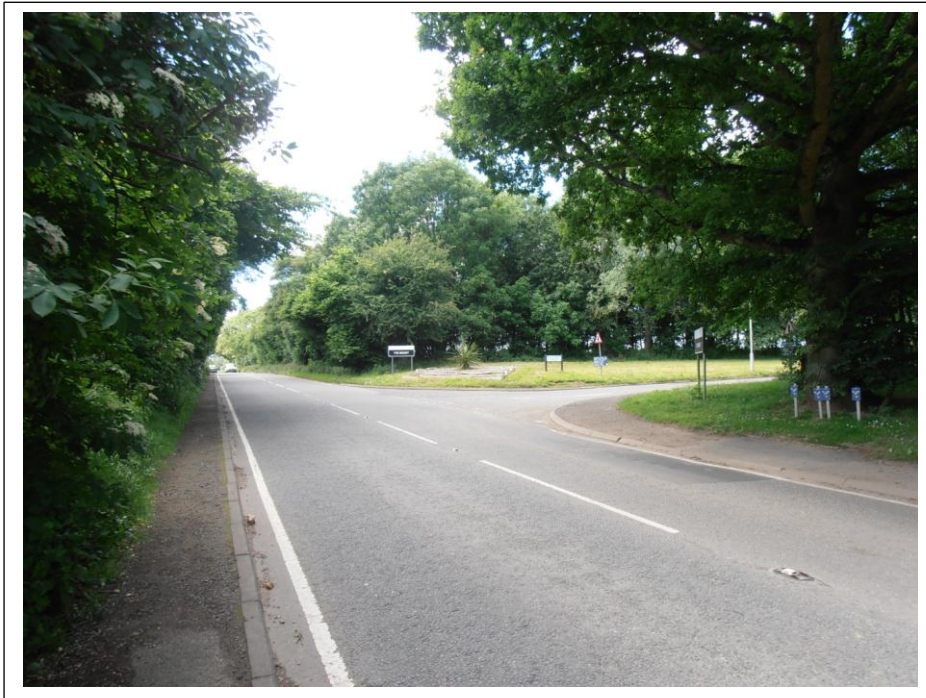
The main site access – off Chesham Road (foreground), via Molyneaux Avenue (right).
