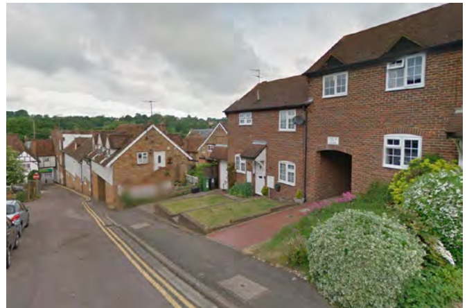
Fig 5.12 The existing homes on the nearby Chapel Street step down the steep hill and provide level access for each dwelling. Front gardens are terraced with the levels of the road.
