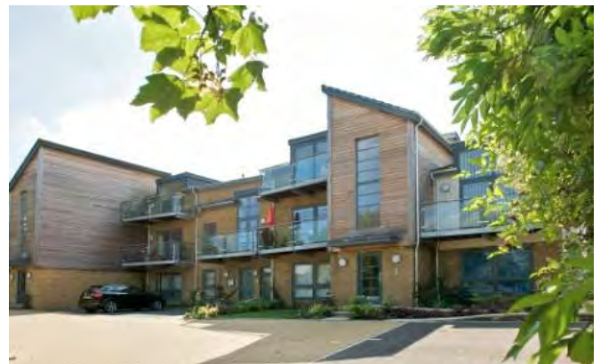
Fig 5.15 Although more modern in style than other examples the articulation of this facade provides opportunities for balconies with privacy from overlooking.
