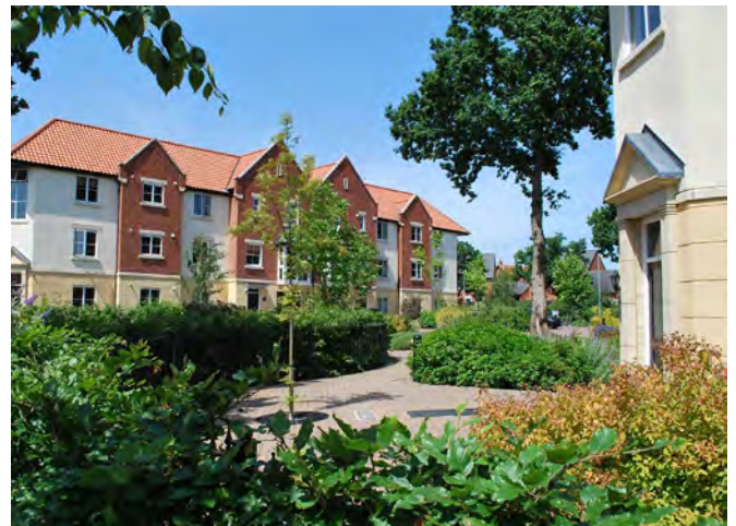
Fig 5.15 The articulation of the elevation of these flats help to break down its overall massing and is also in keeping with the surrounding housing development.
