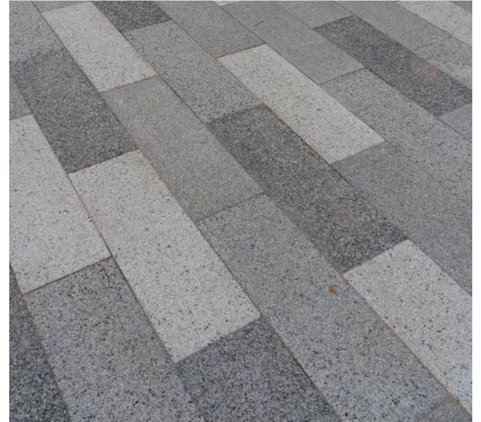
Marlowes Shopping Zone Paving
