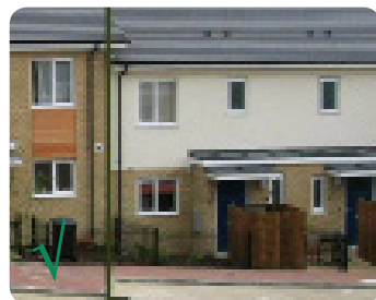
The above example in Hemel Hempstead shows a well ventilated store of an adequate size that has been successfully integrated into the development.
