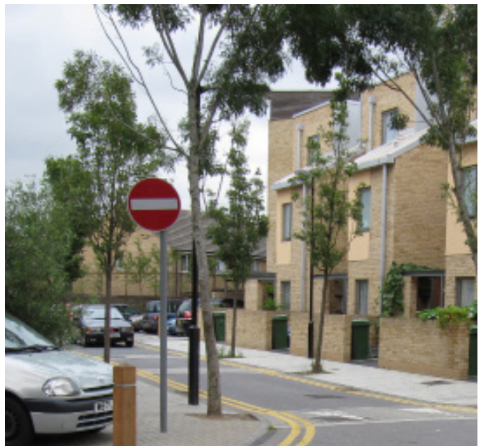
This example shows development at Harmony Place, London. Refuse storage has been integrated into front garden spaces. The design compliments the architecture and screens bins from the street.
