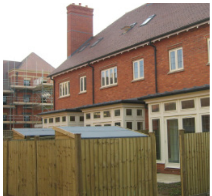
This example shows development at Upton Park. Bin stores have been integrated into back gardens with gate access to a lane for owners to drag their bin to the collection point.
