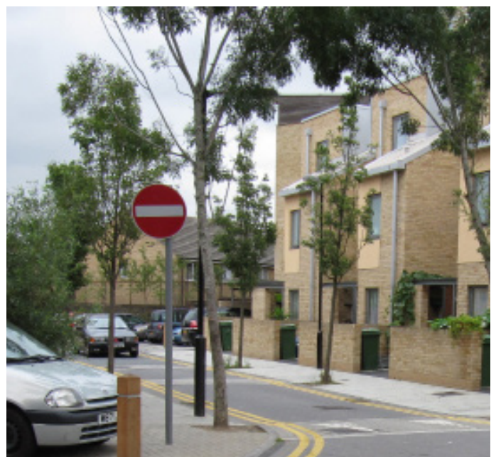
This example shows development at Harmony Place, London. Refuse storage has been integrated into front garden spaces. The design compliments the architecture and screens bins from the street.
