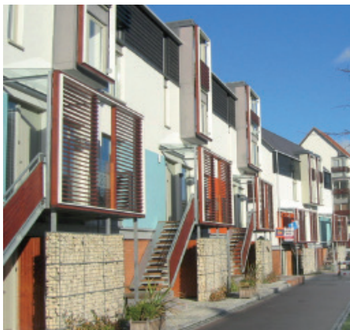
This example shows development at Newhall, Harlow. Space for bins has been cleverly integrated into the facade below the main access to the property.
