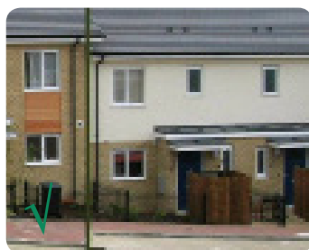
The above example in Hemel Hempstead shows a well ventilated store of an adequate size that has been successfully integrated into the development.
